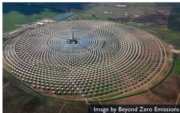
Spain's Gemasolar solar thermal plant uses molten salt storage to run 24 hours per day
