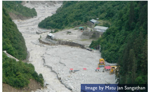
Boulders brought down by the collapse of a mudslide dam created a flash flood in the Bhagirathi River destroying the Vishnuprayag power station in Uttarakhand, India. June, 2013
