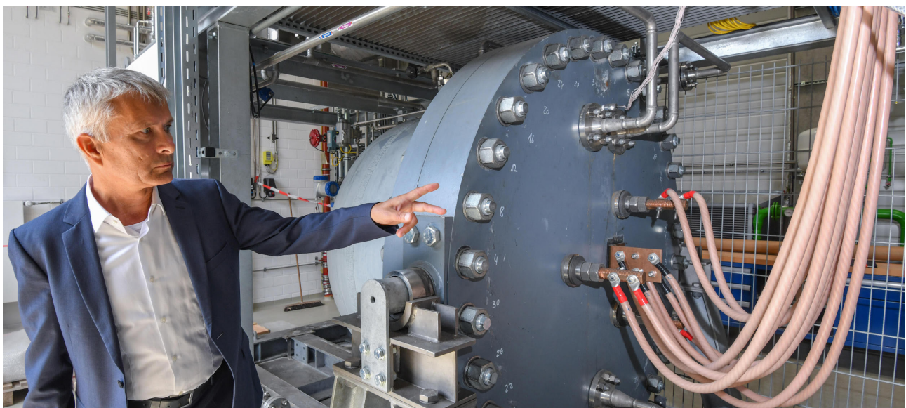
An alkaline pressure electrolyser, used in the production of hydrogen, at the Hydrogen Research Centre of Brandenburg Technical University, Germany. (Image: Alamy)
