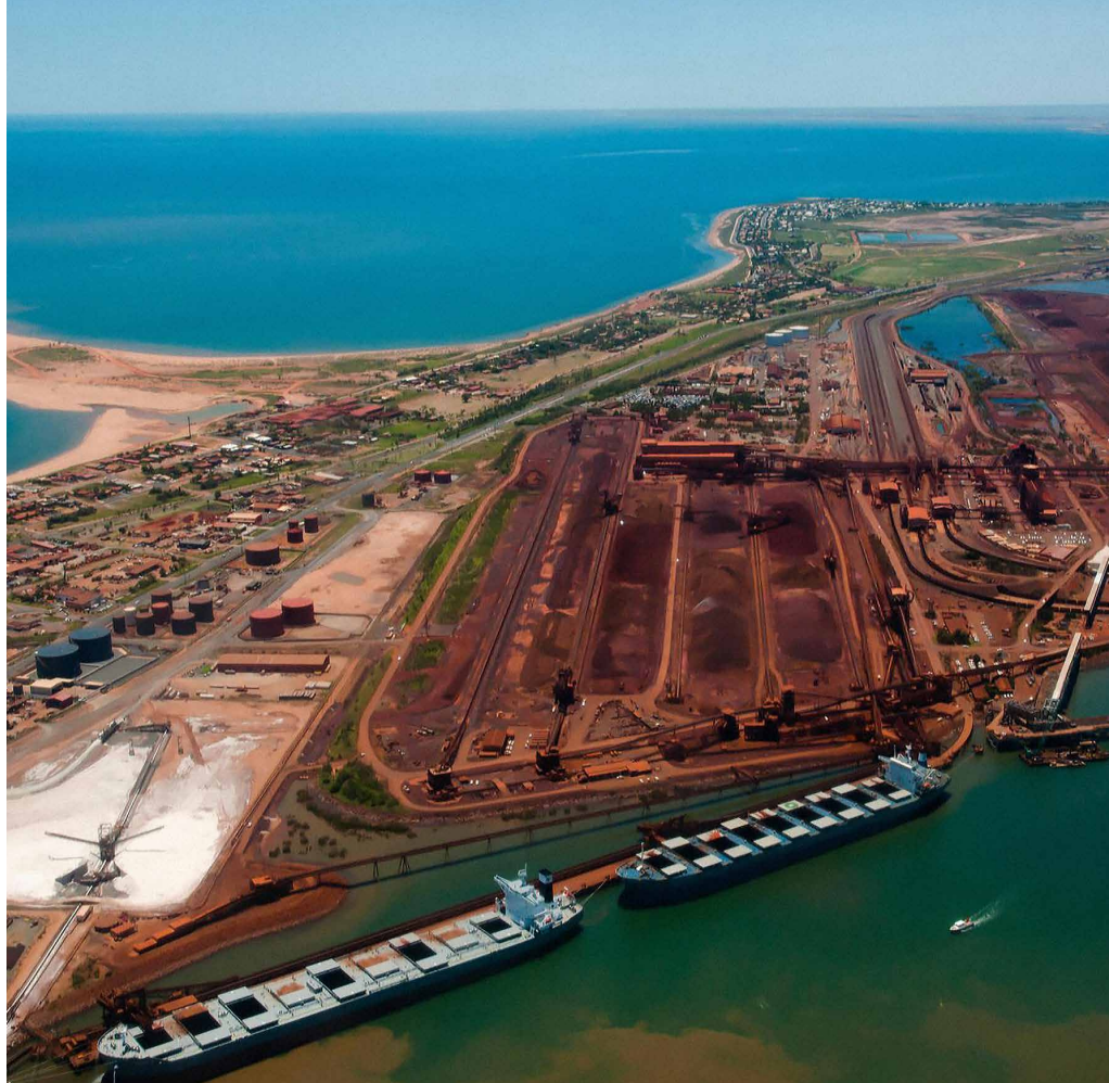
Sixty-five million tonnes of iron ore are exported between Australia and Japan each year. Australia is investing heavily in hydrogen production capacity, much of it near major ports such as Port Hedland. (Image: Adrian Wojcik / Alamy)
