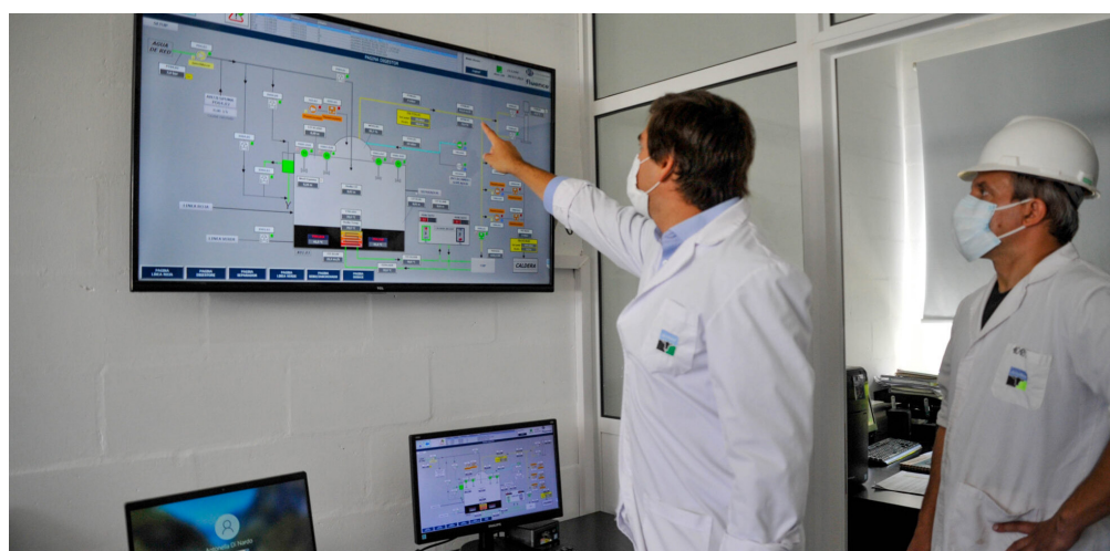
Plant manager Mauricio Accietto explains how bacteria inside the biodigester decompose organic waste to create biogas, which is then fed into the facility's generator. In 2021, only 13% of Argentina's energy came from renewable sources, with bioenergy accounting for just 6% of this renewable generation. Image: Celina Mutti Lovera / Diálogo Chino
