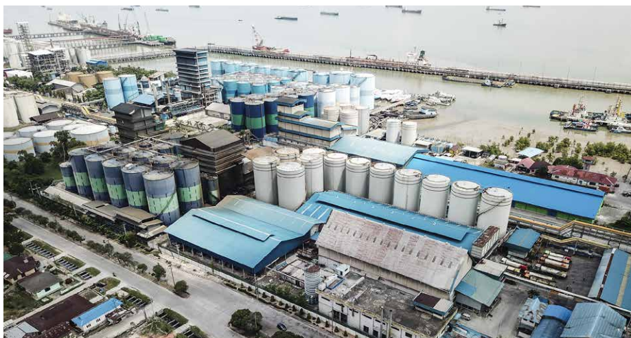
Wilmar International's palm oil refinery in Dumai, Sumatra. Most of a refinery's greenhouse gas emissions come from the energy needed to power its operations. (Image: Wahyudi / China Dialogue)
